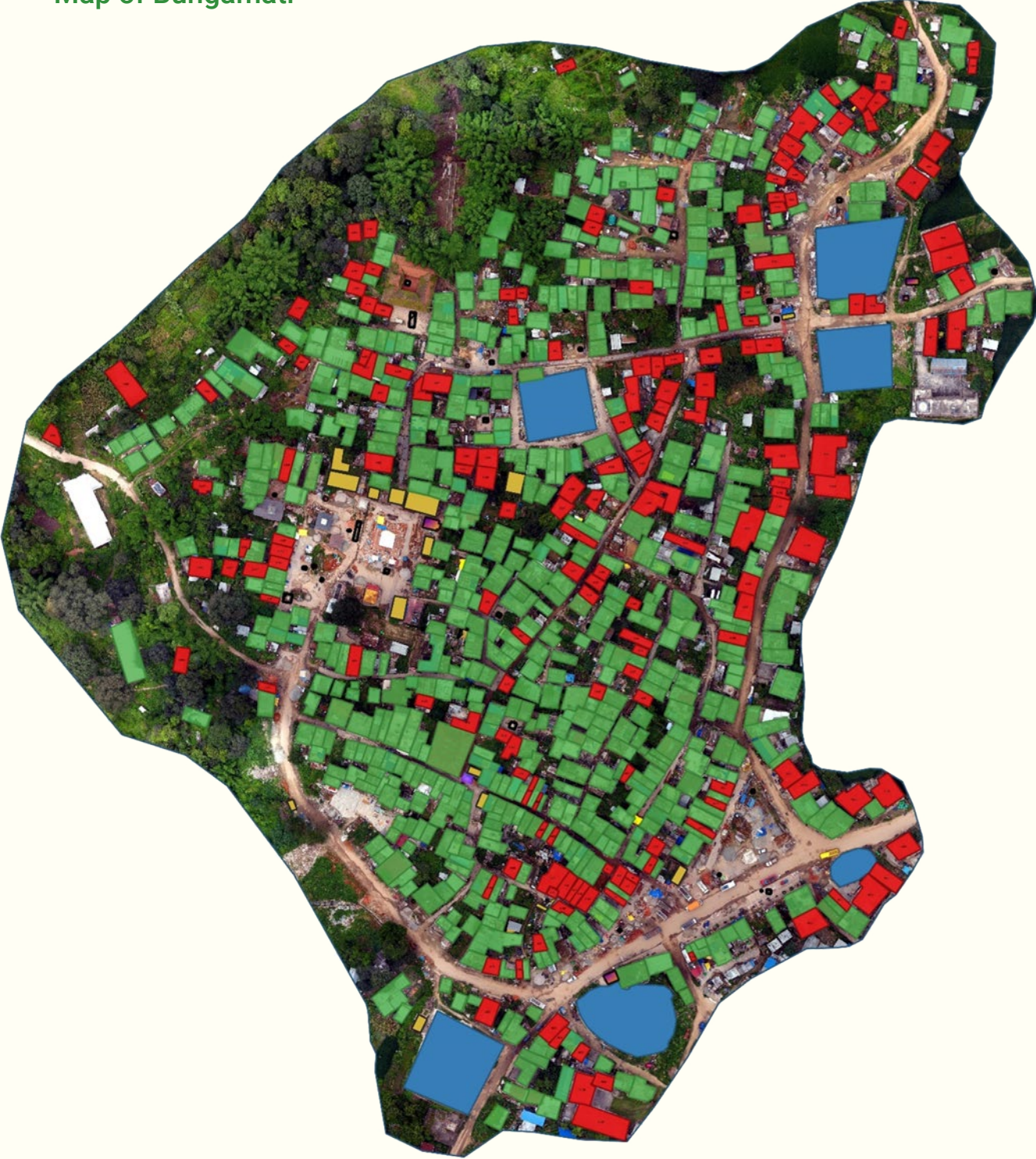
Fig: Aerial Map showing the existing condition of the of the core settlement of Bungamati as of June 2018. The Green roofs indicate the houses and the red are the temporary shelters constructed after the earthquake.
